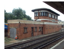
Woking Signal Box Finished in 1937 it is an example of the Art Deco style. It stopped being used as a signal box in 1997 but cannot be knocked down.
